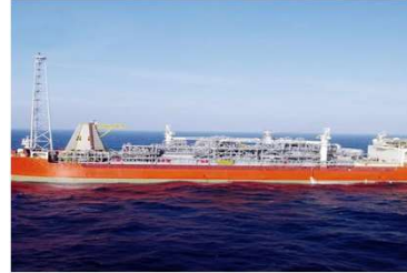
Offshore Texaco Captain Production Platform
