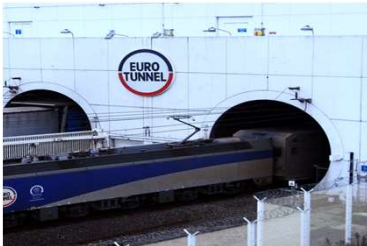
Construction Channel Tunnel France to UK
