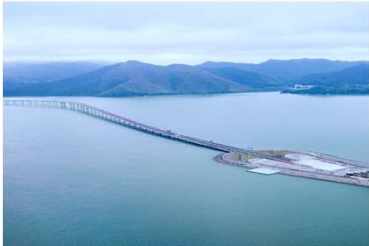
Construction Hong Kong Macao Bridge
